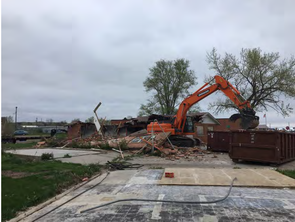
Building demolition to expose sub-slab transite pipe.
