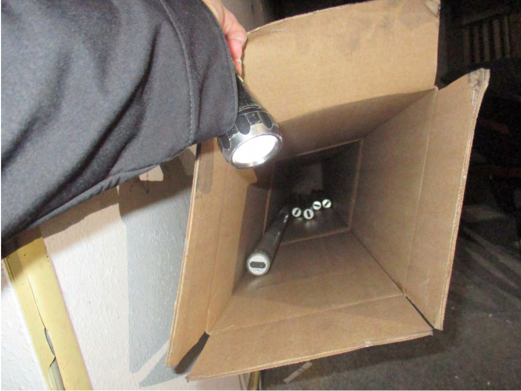
Only 5 fluorescent bulbs were found in the structure. These were recycled.
