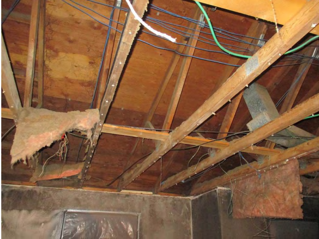
Ceiling removal was completed throughout the interior.
