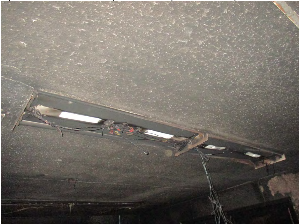
Fluorescent bulbs and ballasts were removed.
