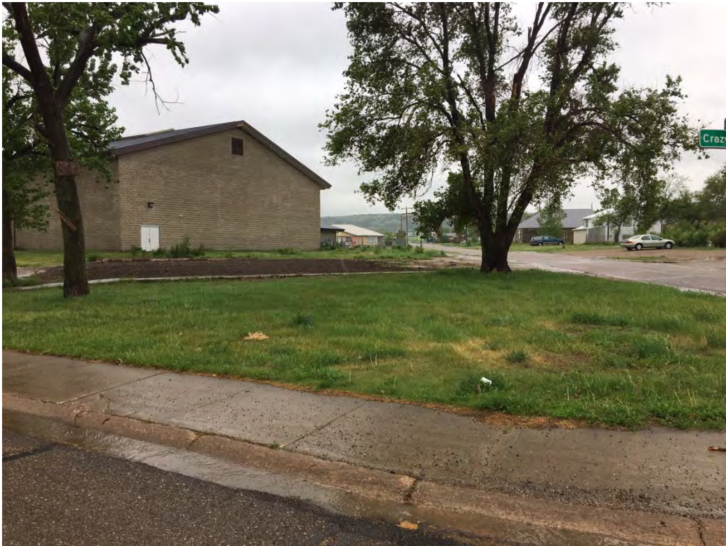
Topsoil placed and graded
