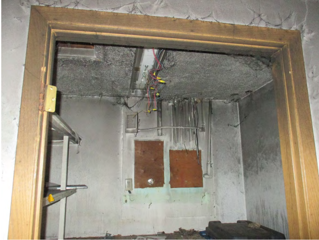
Electrical panels were removed by vandals prior to hazardous materials removal.
