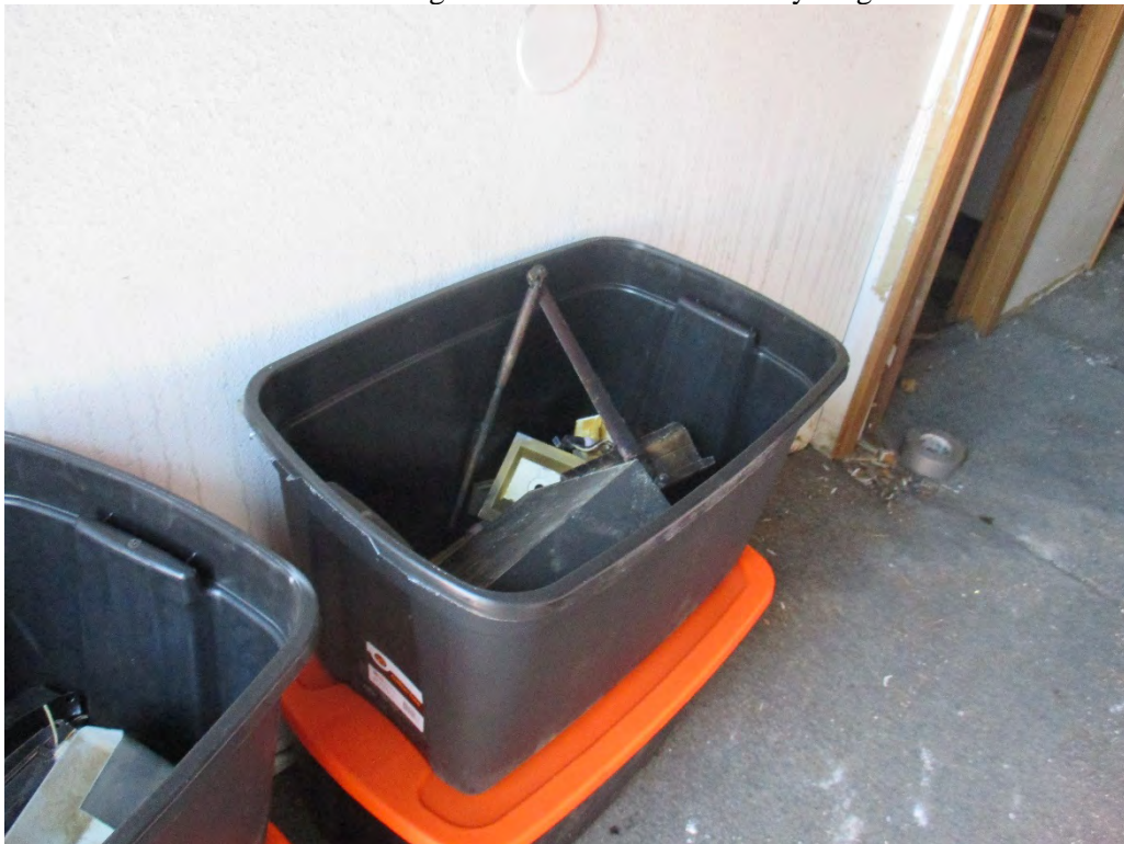
Exit signs and door closers. Exit signs were recycled. Door closers were opened and did not contain oil. The door closers were disposed as regular solid waste.
