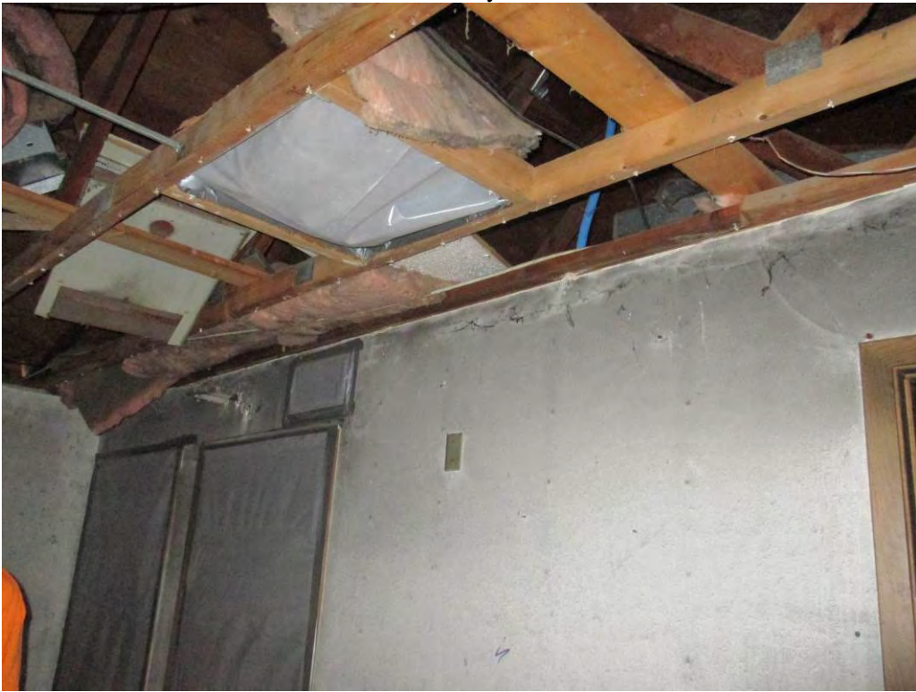
The water line with ceiling texture overspray was fully removed.
