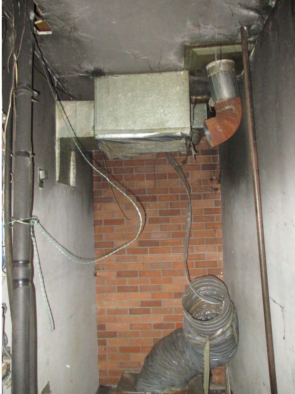
The furnace was removed by vandals prior to hazardous materials removal.
