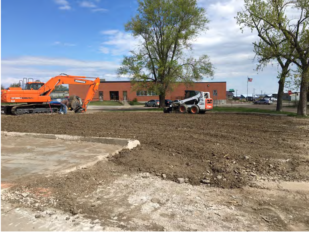
Final grading of topsoil
