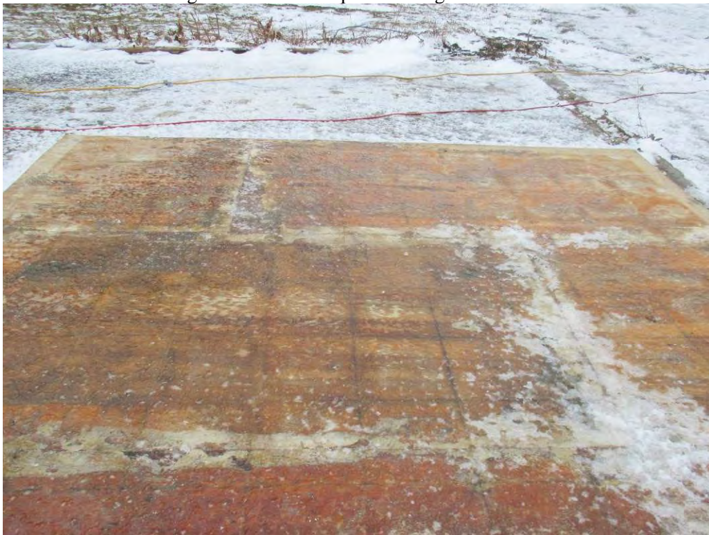
Floor tile removal on the exterior slab. The mastic was not asbestos containing.
