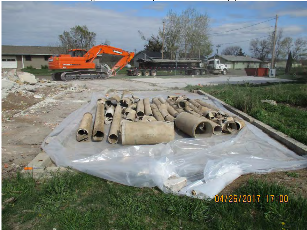
Transite pipe removal.
