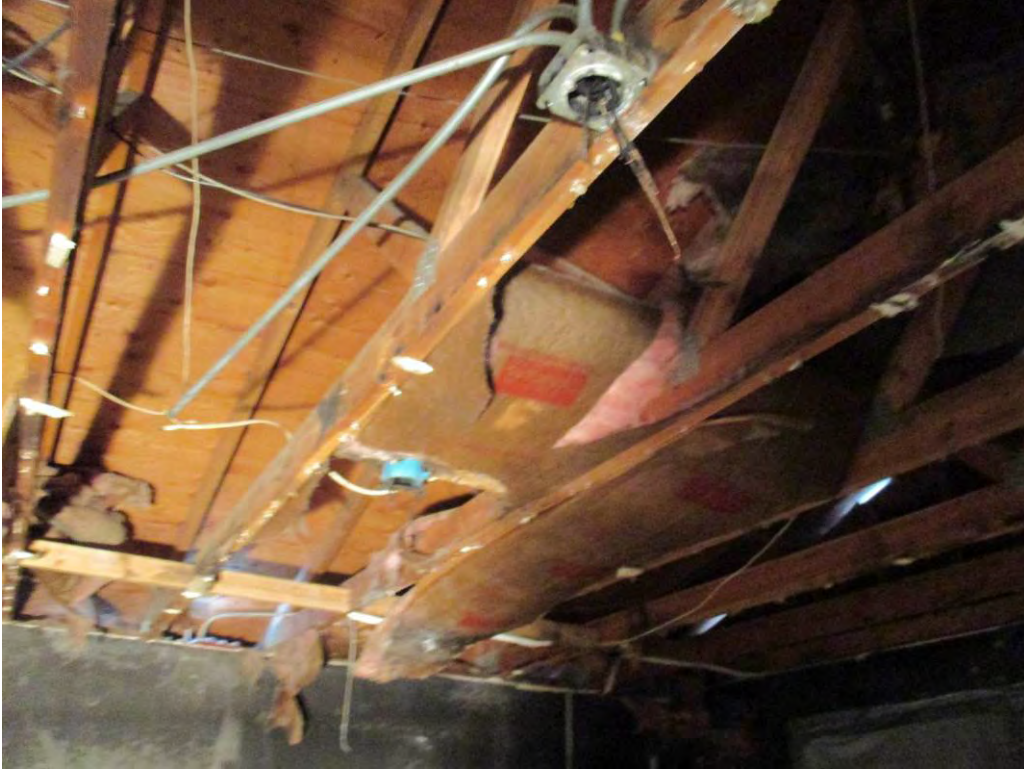
Ceiling texture removal (typical). Texture was well adhered and full ceiling removal was more time efficient than texture-only removal.
