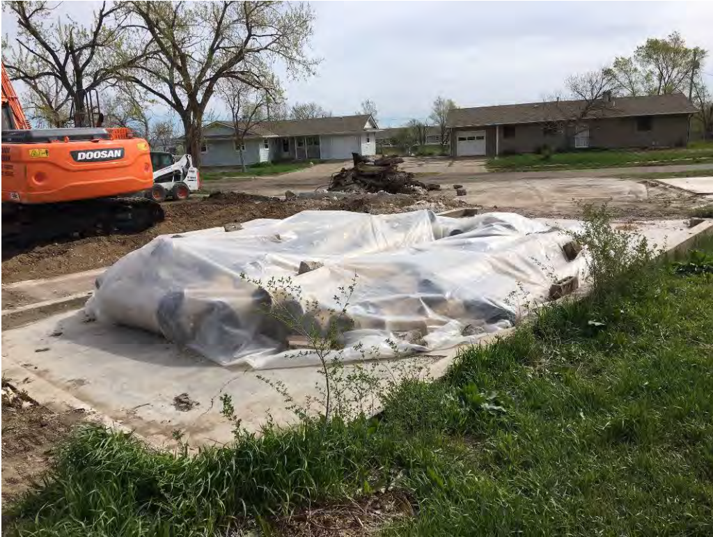
Transite pipe wrapped in preparation for collection and disposal.
