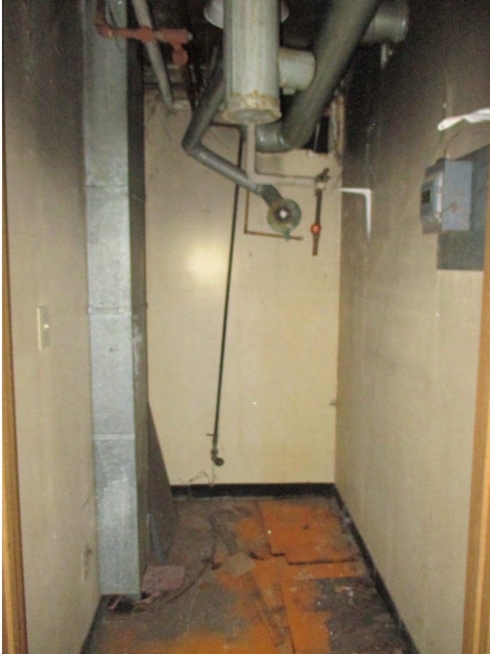
The water heater was removed by vandals prior to hazardous materials removal.
